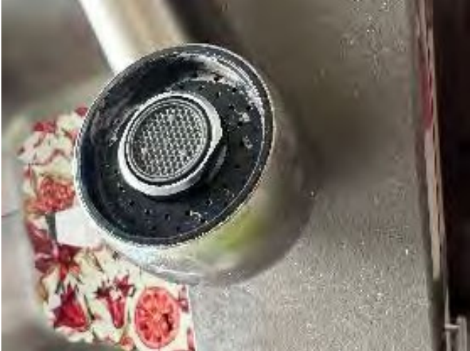
Photograph 1: Exterior of Kitchen faucet aerator. Note that there are small white particles on the exterior of the aerator.
