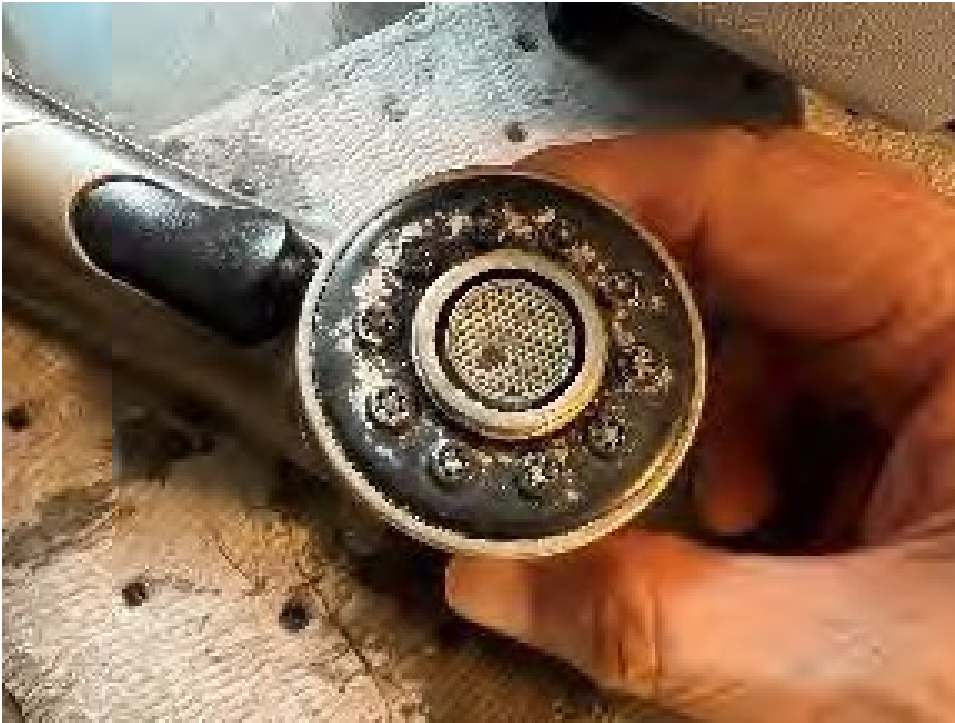
Photograph 2: Exterior of Kitchen faucet aerator, with a few small particles and scaling.
