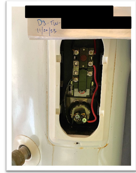
2023.11.20 / ADDRESS G Water Heater Thermostat
