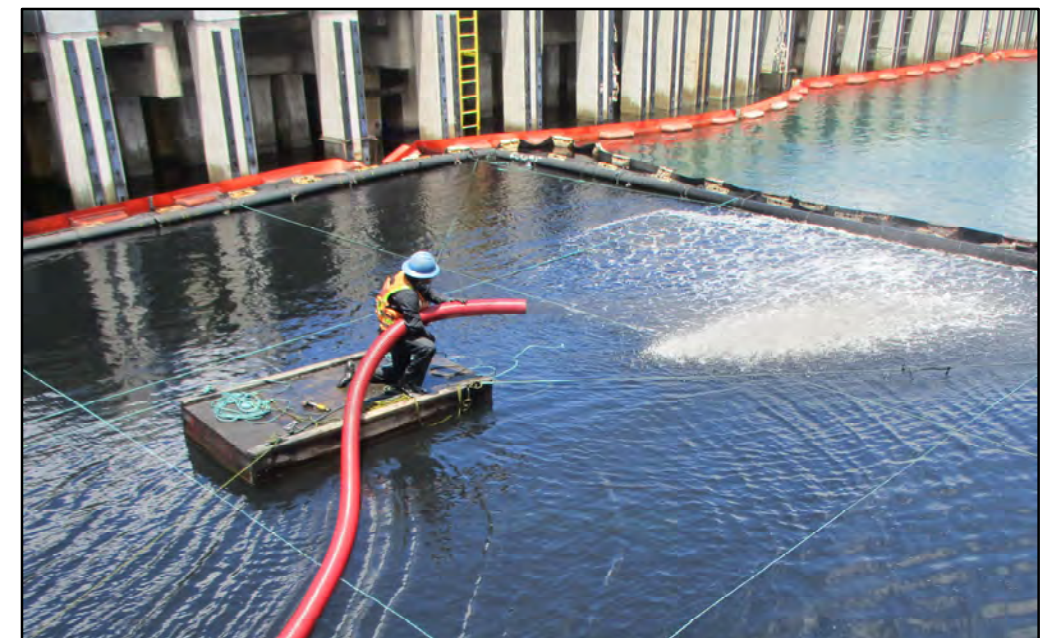
AC material delivery in overwater treatment area
