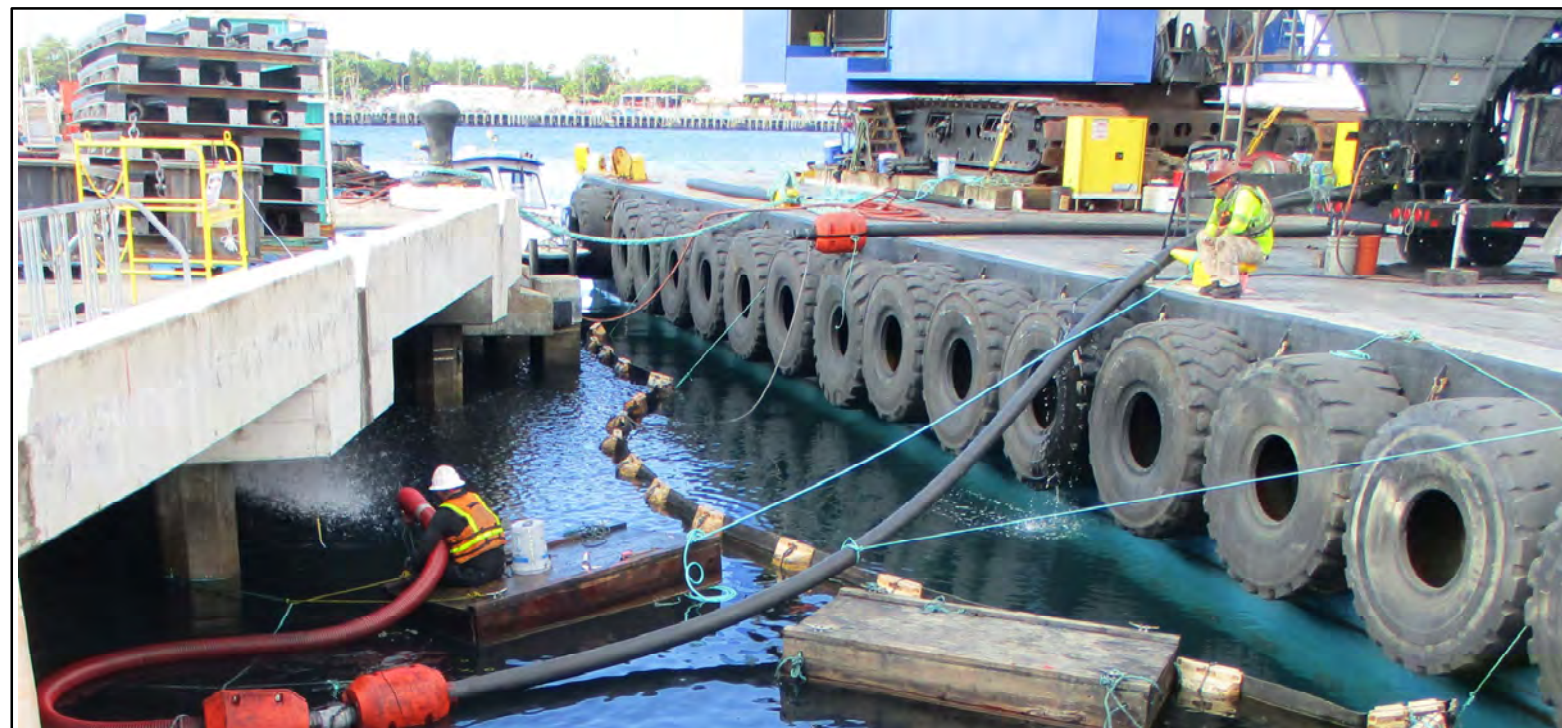
AC material delivery in under pier treatment area
