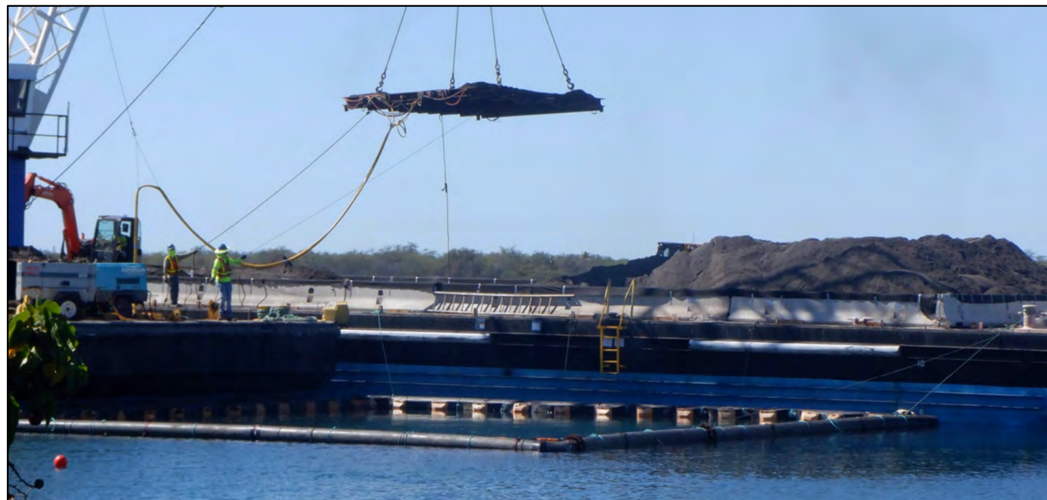
Sand placement box suspended over delivery cell
