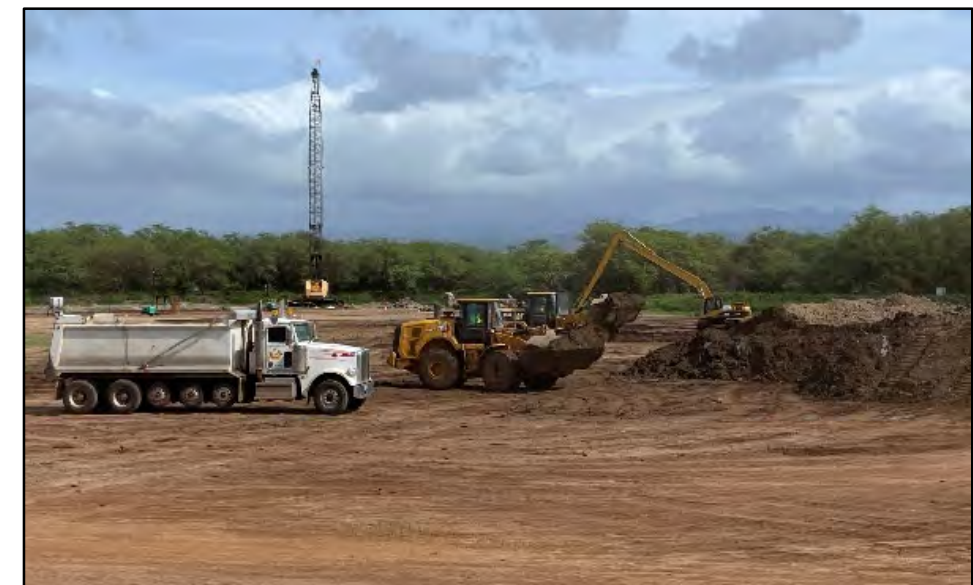
Dredged material loading for transport to disposal facility
